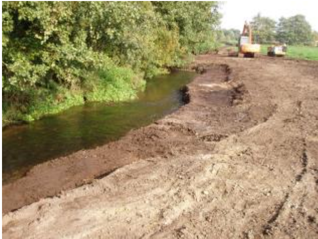
Spoil bank removal, October 2006
