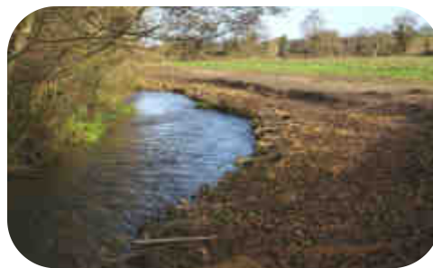
Profiling work finished
