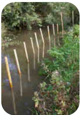
Preparation for river narrowing and finished work showing new profile of river.
