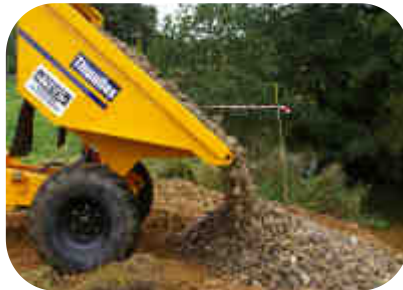
Construction of cattle crossing and riffle
