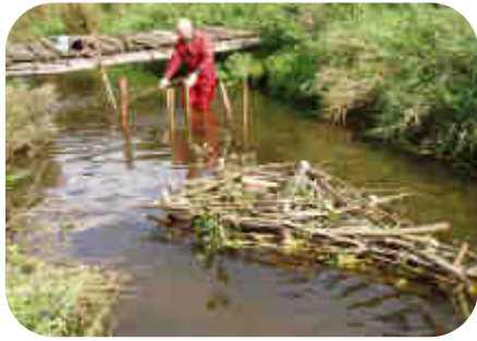
Construction of mid stream islands, completed islands and riffle constructed around them
