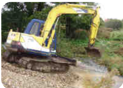
Construction of cattle crossing and riffle
