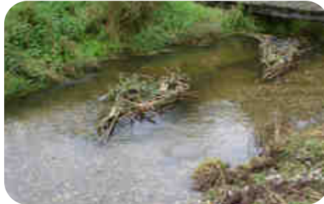
Construction of mid stream islands, completed islands and riffle constructed around them
