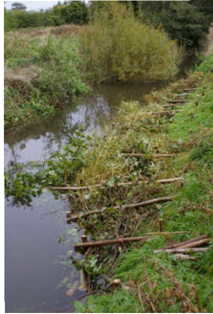
River narrowing 1; opposite two willows, one coppiced to contribute to back-fill. [05/10]
