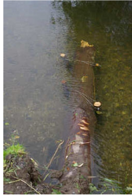
Staking and fencing wire support for LWD [06/10]
