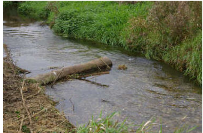
LWD 5 on riffle 5, showing flow deflection [16/10]
