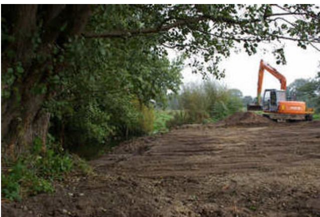
Digger working on final (downstream) stretch of spoil removal [16/10]
