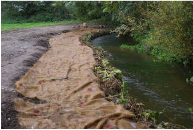
Bank protection, upstream section [25/10]
