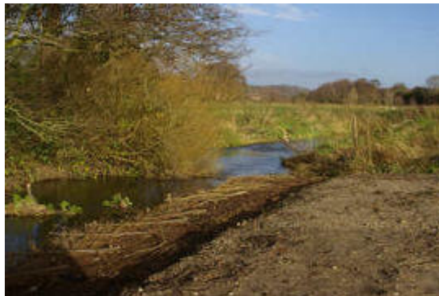
Close up of bank protection, which was finished with the coir matting to prevent soil loss in flood and will allow vegetation to grow through. Also shows LWD 9 and cattle crossing 3; latter done by hand with recovered stone and "gleaned" gravel [07/12]
