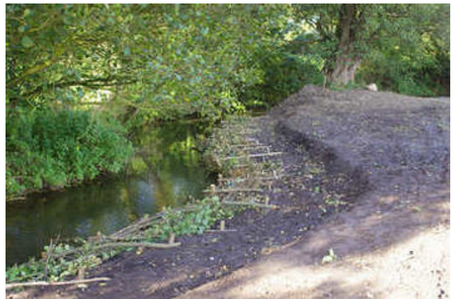
Bank protection around the old alder, tree 1 [21/10]
