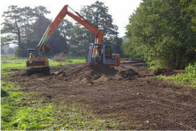
Spoil removal by tracked digger and 2 dumpers working in tandem [11/10]
