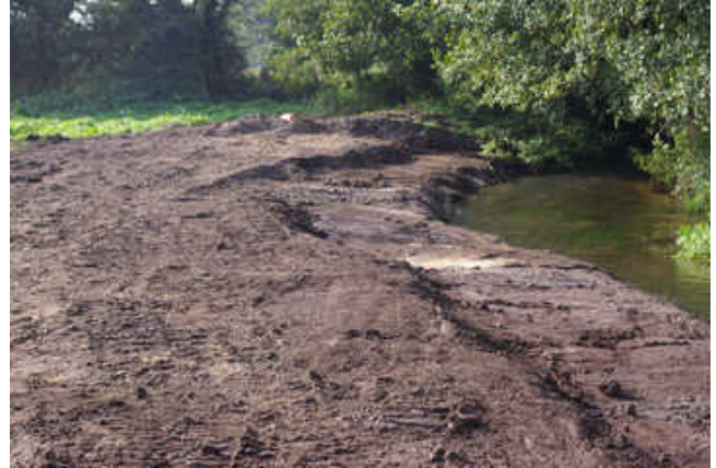
Re-profiled river bank, upstream end [11/10]
