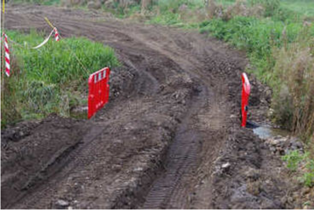
Temporary bridge across side channel, installed 11/10 after a shower of rain [16/10]
