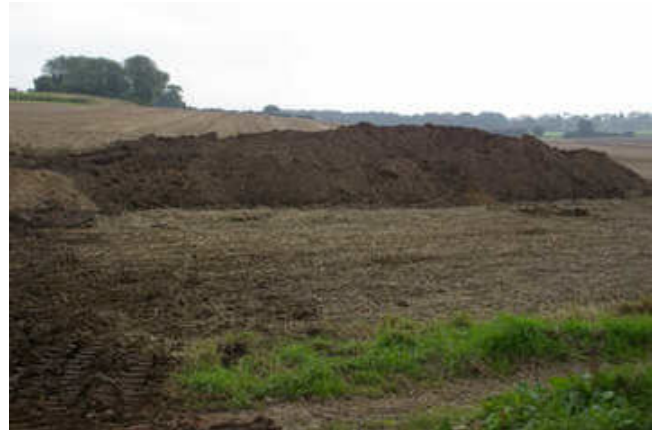
Spoil was deposited on arable field. Large stone was removed by hand either at meadow or field end [16/10]
